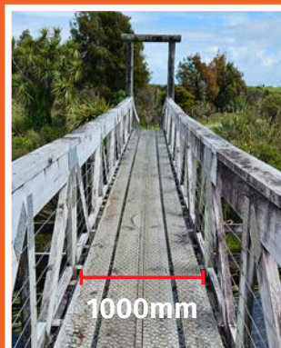
Mahinapua Creek bridge
