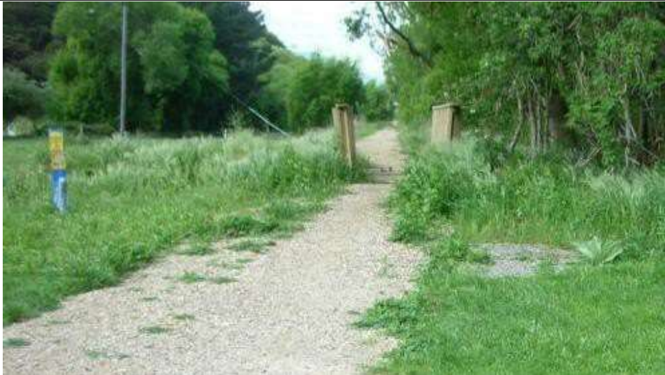
Figure D4: Compacted gravel section of Little River Rail Trail at Catons Bay
