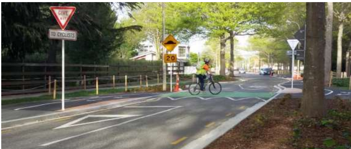
Figure 67: Supplementary ‘to cyclists’ plate on give way sign at midblock priority cycle crossing, Uni-Cycle route, Christchurch
