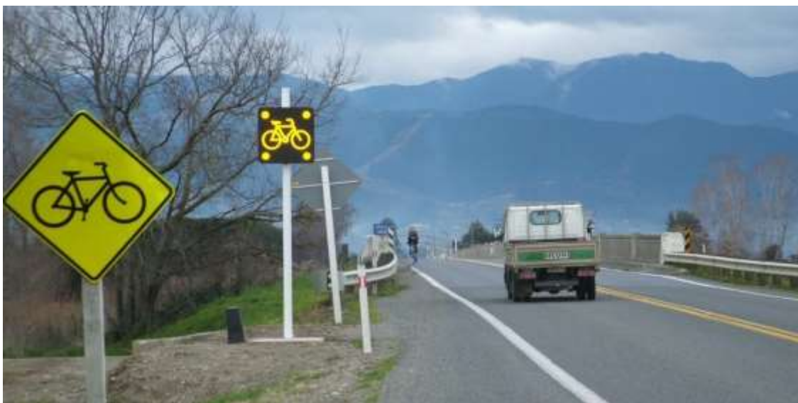
Figure 24: Inductive loop activated warning sign on Appleby bridge, SH 60, near Nelson (Photo: NZTA)
