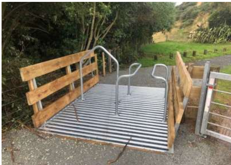
Figure E11: Example of a wheelchair-accessible barrier, Belmont Regional Park (Photo: Greater Wellington Regional Council)
