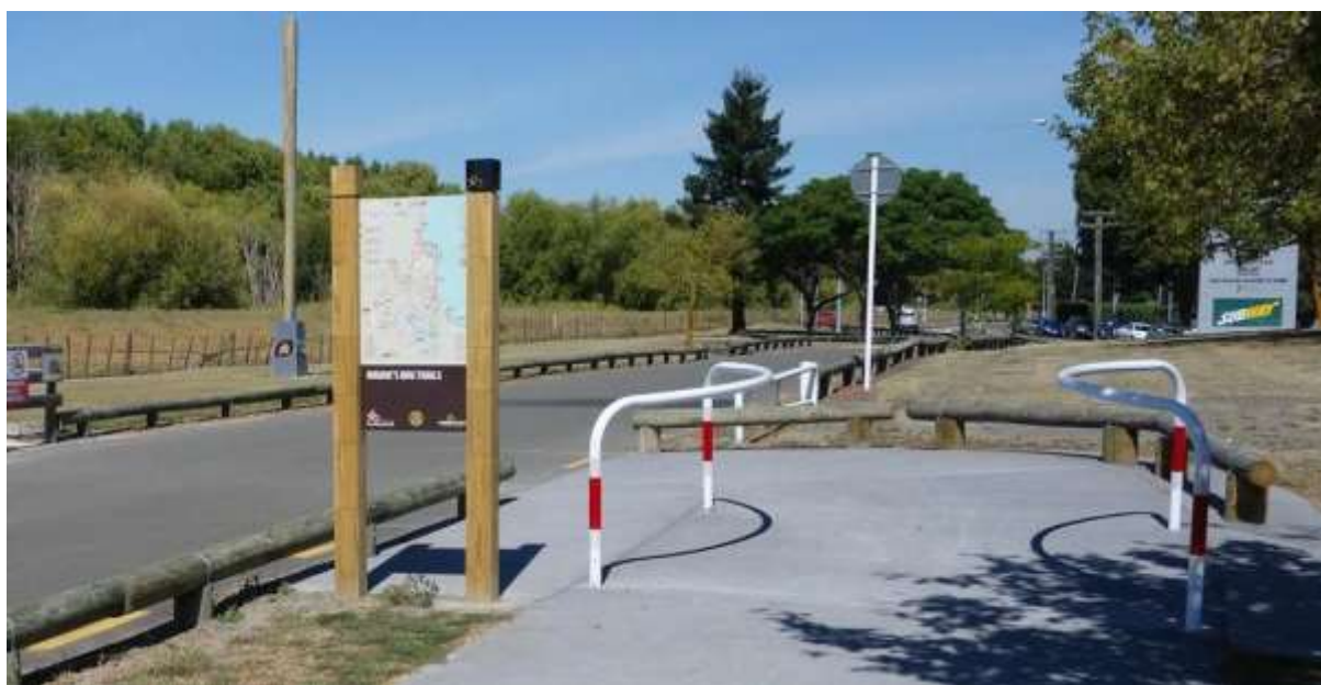
Figure B16: Path end treatment, Hawkes Bay Trails (Photo: Jonathan Kennett)
