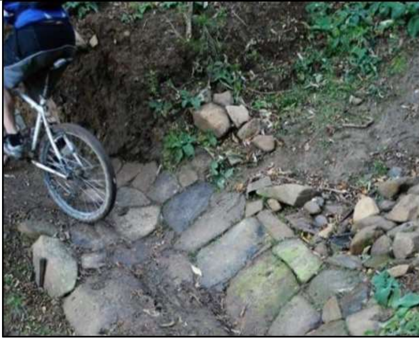
Figure C7: Rock armoured path – Nichols Creek Track, Dunedin (Photo: Kennett Brothers)
