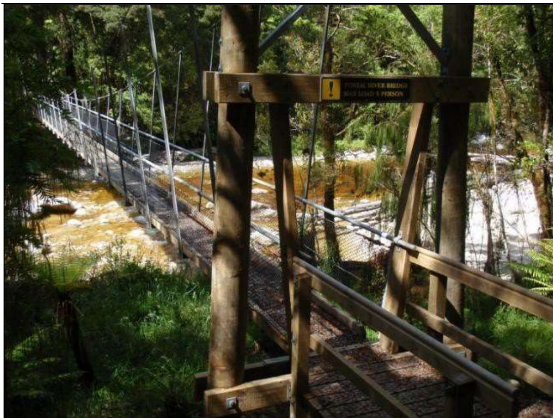
Figure D17: Suspension bridge, Ōparara Valley Track
