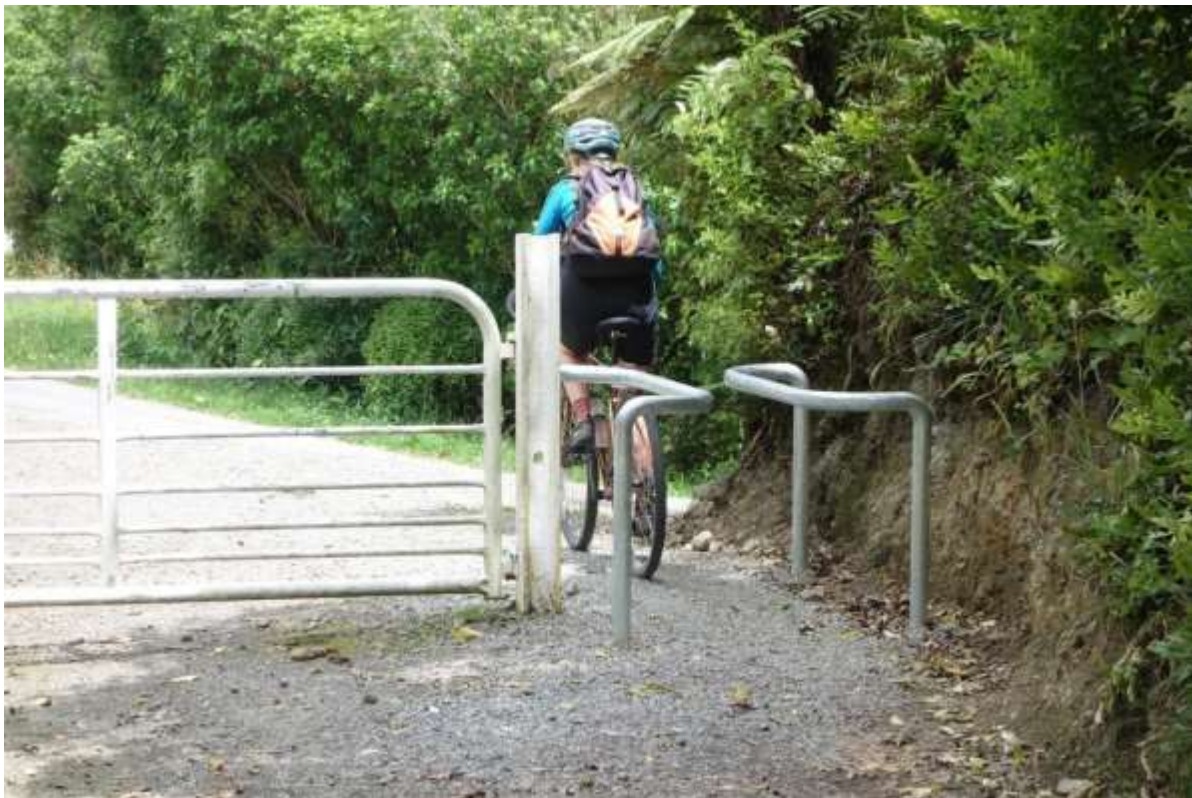
Figure E14: ‘Squeeze barrier’ to discourage motorcycles, Remutaka Cycle Trail (Photo: Jonathan Kennett)
