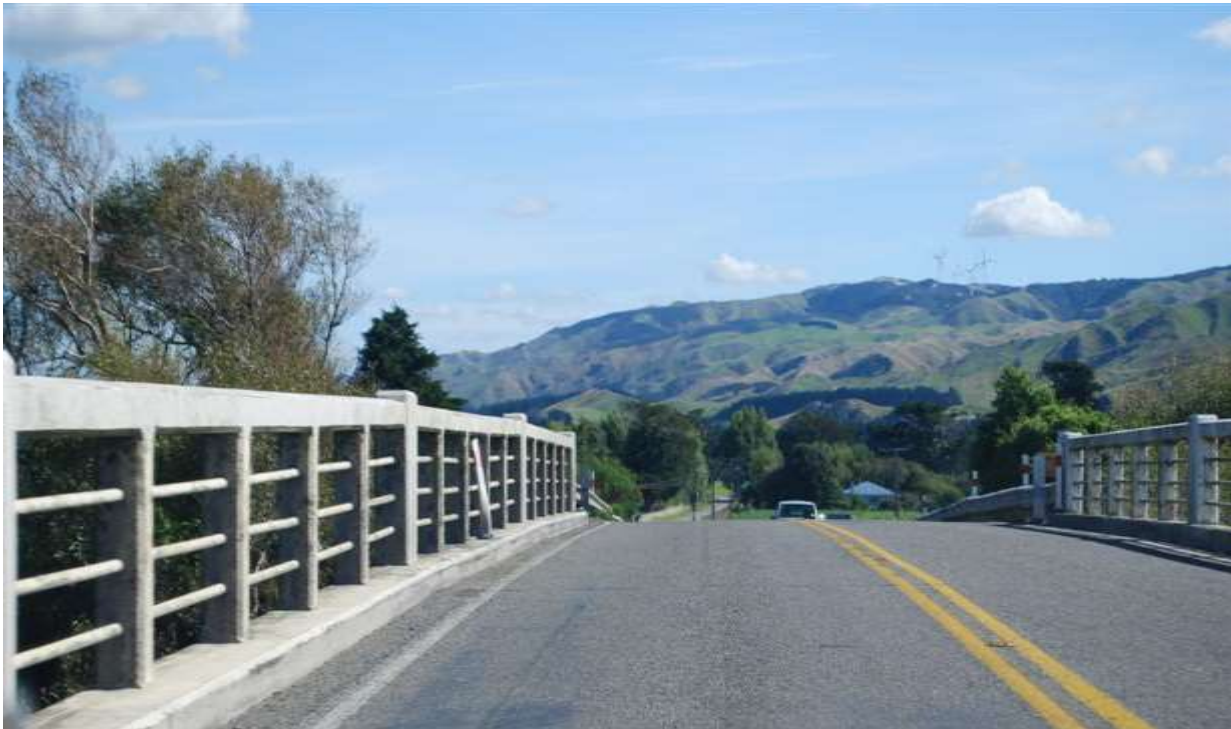
Figure 33: Many railway over-bridges have inadequate shoulder width and may require clip-on bridges on each side for cycling safety (Photo: Jonathan Kennett)
