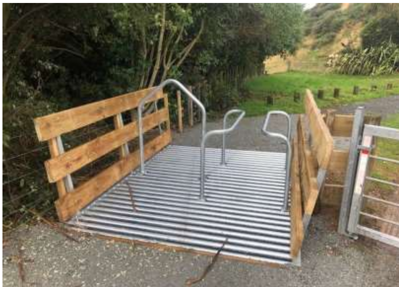
Figure D11: Example of a wheelchair-accessible barrier, Belmont Regional Park (Photo: Greater Wellington Regional Council)
