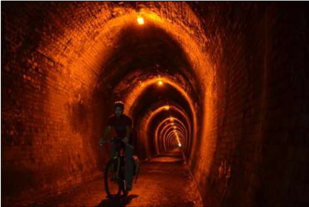
Figure 42: Tunnel on the Hauraki Rail Trail (Photo: Jonathan Kennett)
