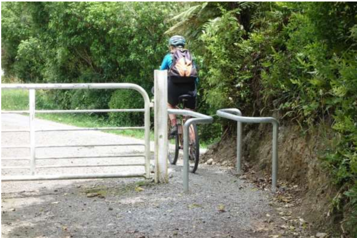
Figure B17: 'Squeeze barrier' to discourage motorcycles, Remutaka Cycle Trail (Photo: Jonathan Kennett)
