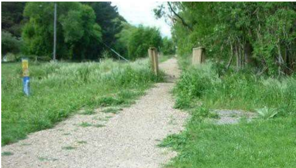
Figure E4: Compacted gravel section of Little River Rail Trail at Catons Bay
