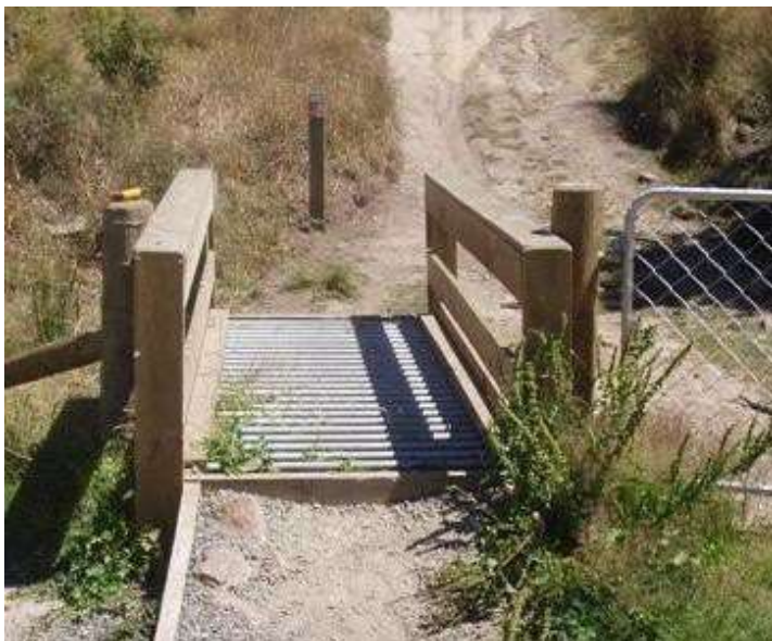
Figure 38: Cattle stop with good alignment, Port Hills (Photo: Nick Singleton)
