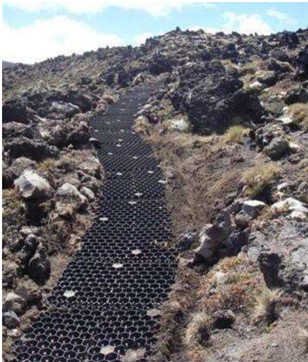
Figure A5: 'Geomat' surface stabilisers (prior to having aggregate placed on top), Tongariro National Park (Photo: John Bradley)
