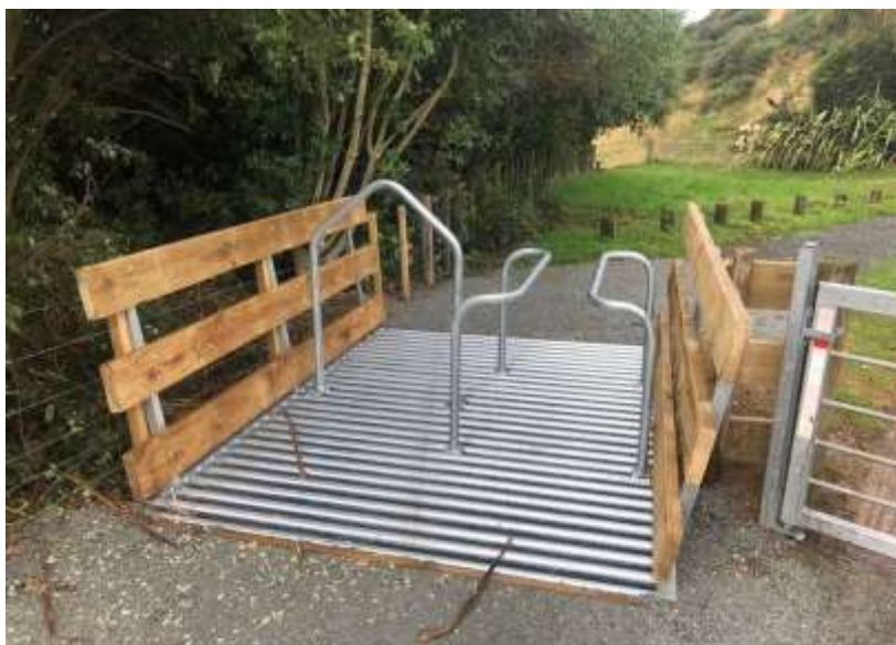
Figure C11: Example of a wheelchair-accessible barrier, Belmont Regional Park (Photo: Greater Wellington Regional Council)
