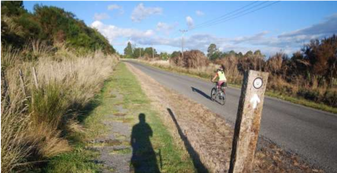
Figure 6: Poorly surfaced cycle paths next to low-volume roads will not be used by cyclists
