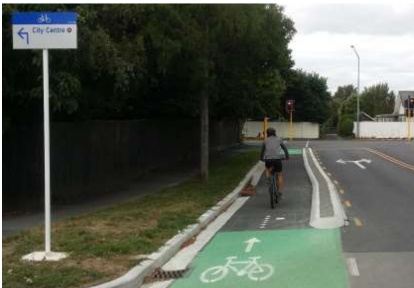
Figure 3: Separated paths on Rutland Street, Christchurch
