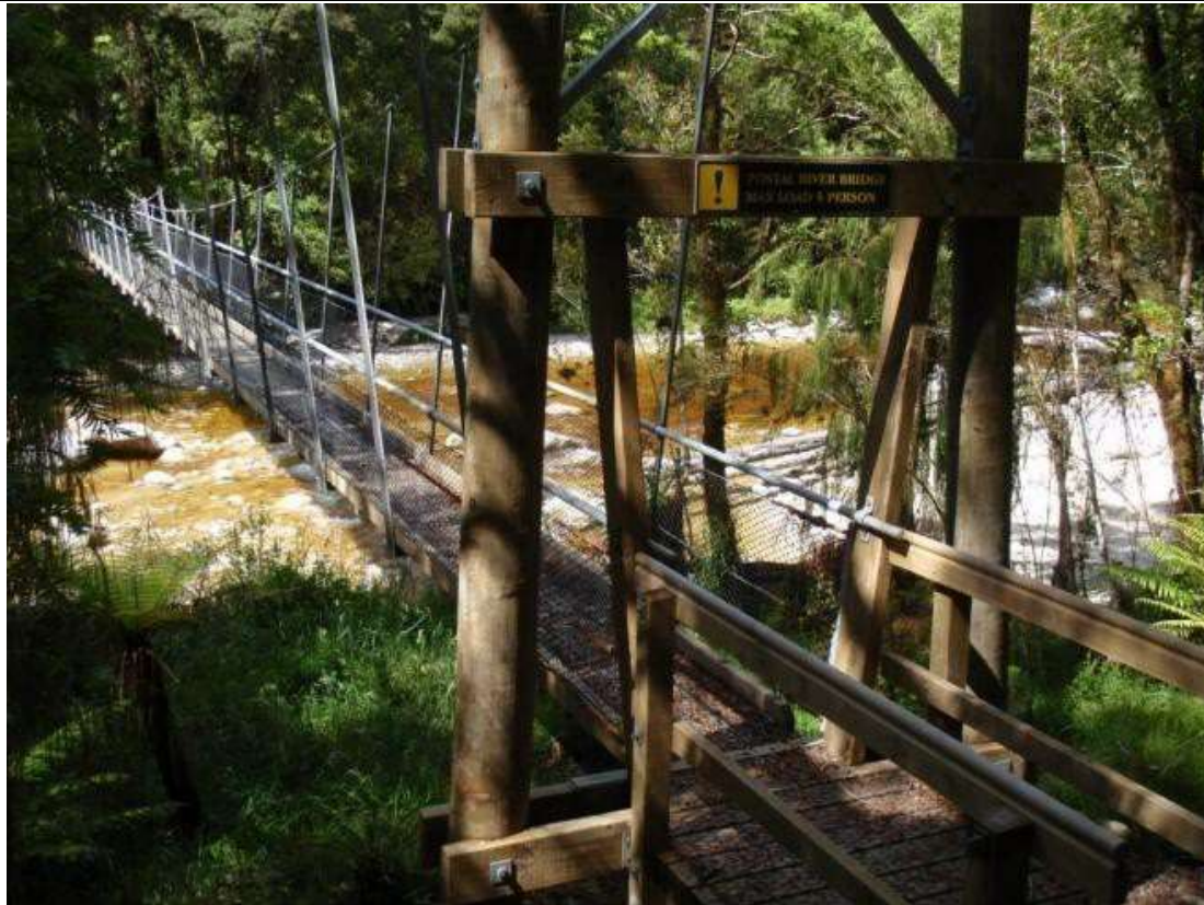
Figure C17: Suspension bridge, Ōparara Valley Track
