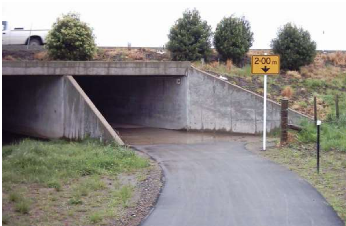
Figure A2: Warning sign for a low underpass, Nelson
