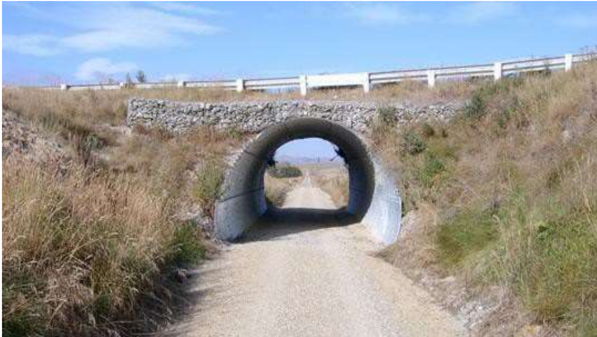
Figure 29: Otago Central Rail Trail underpass (Photo: courtesy of OCRT Trust)
