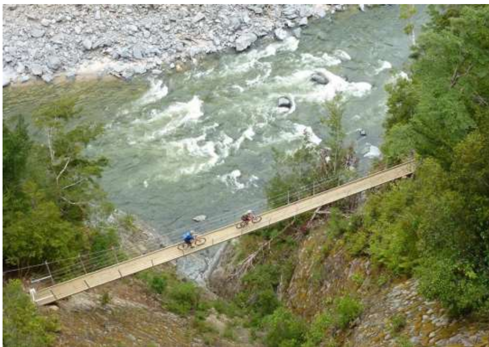
Figure B19: Suspension bridge on the Old Ghost Road (Photo: Jonathan Kennett)
