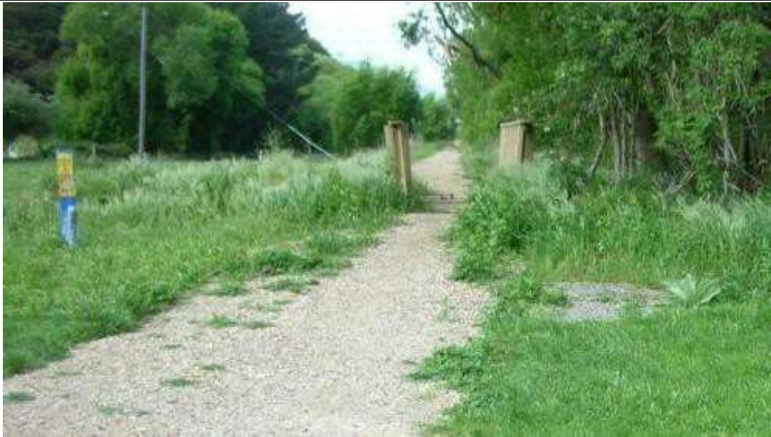
Figure A4: Compacted gravel section of Little River Rail Trail at Catons Bay
