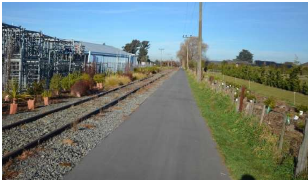
Figure A9: Asphaltic concrete path on the Little River Rail Trail (Photo: Jonathan Kennett)
