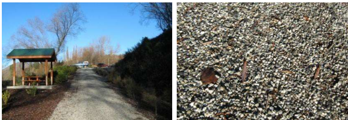
Figure B7: Chip seal path in Queenstown
