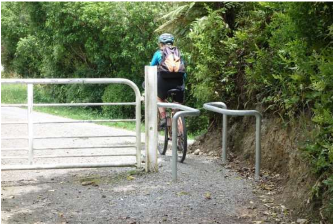
Figure A17: 'Squeeze barrier' to discourage motorcycles, Remutaka Cycle Trail (Photo: Jonathan Kennett)
