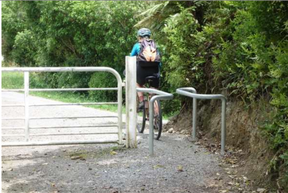
Figure C14: 'Squeeze barrier' to discourage motorcycles, Remutaka Cycle Trail (Photo: Jonathan Kennett)
