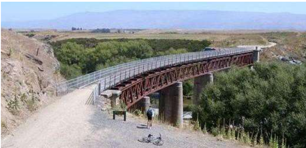
Figure 34: Manuherikia Bridge, Otago Central Rail Trail (Photo: DOC)
