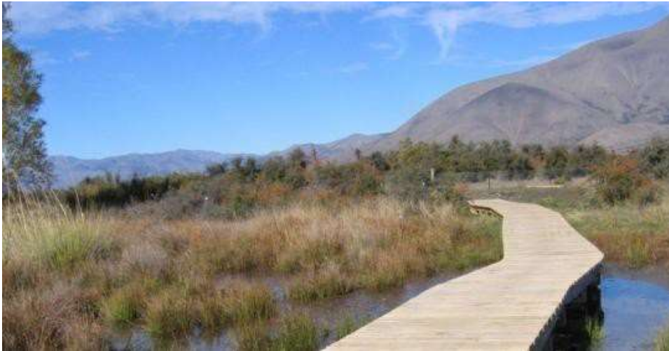
Figure C15: Boardwalk – Twizel River Trail (Photo: Kennett Brothers)
