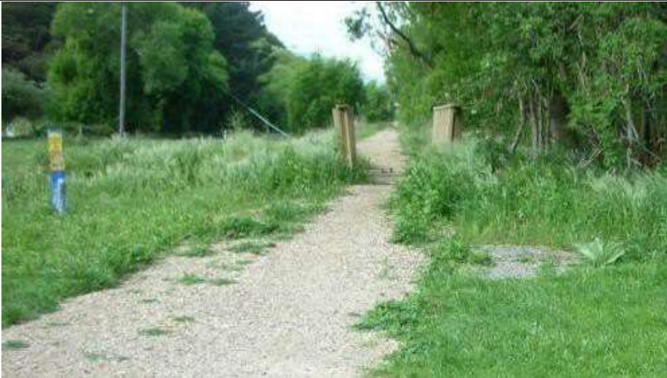
Figure B4: Compacted gravel section of Little River Rail Trail at Catons Bay
