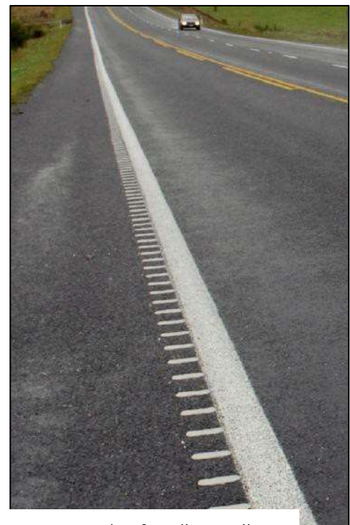
Figure 27: Example of audio-tactile profile (ATP) markings outside an edge-line
