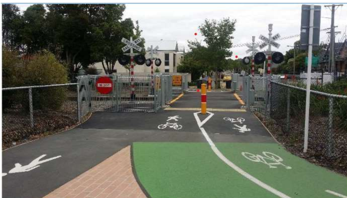
Figure A11: Transition between shared path, footpath and separated cycleway, Matai Street, Christchurch
