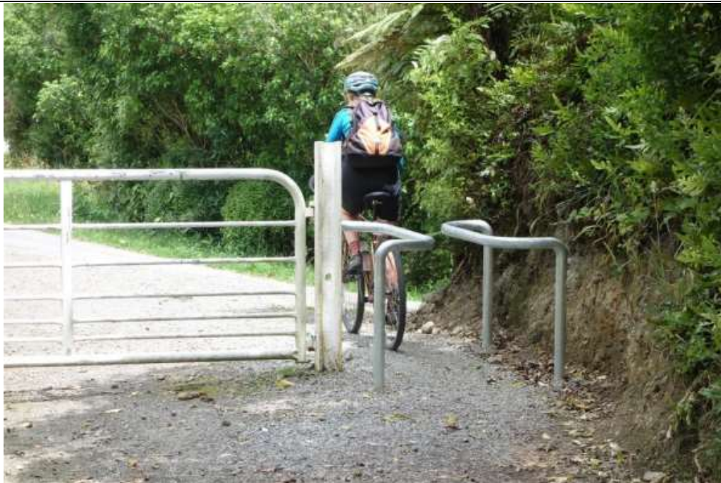
Figure D14: 'Squeeze barrier' to discourage motorcycles, Remutaka Cycle Trail (Photo: Jonathan Kennett)
