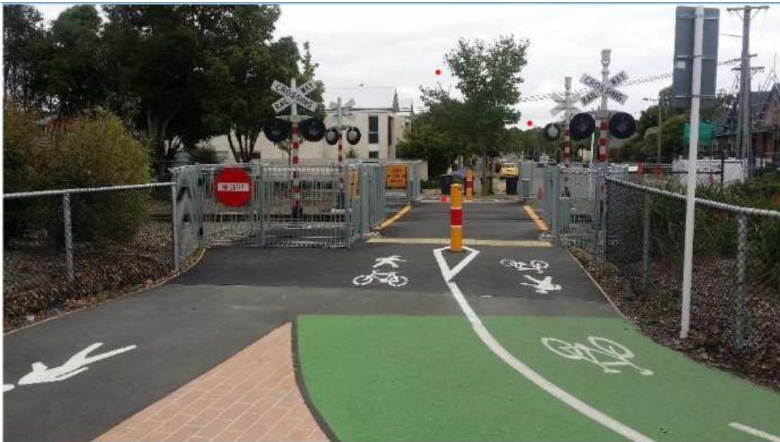
Figure B11: Transition between shared path, footpath and separated cycleway, Matai Street, Christchurch
