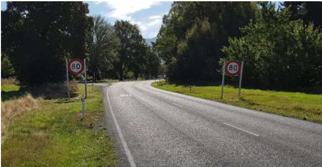
Figure 15: Gated 80 km/h speed limit signs, near Fairlie
