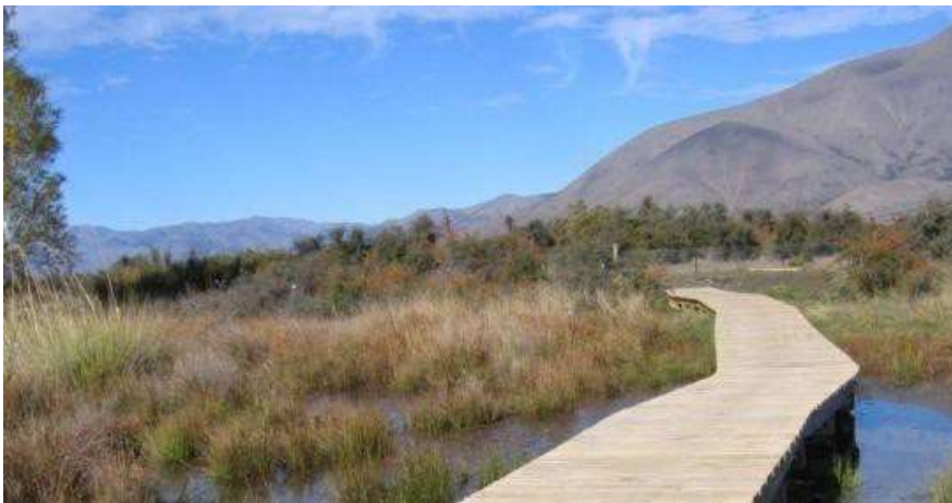
Figure B18: Boardwalk – Twizel River Trail (Photo: Kennett Brothers)
