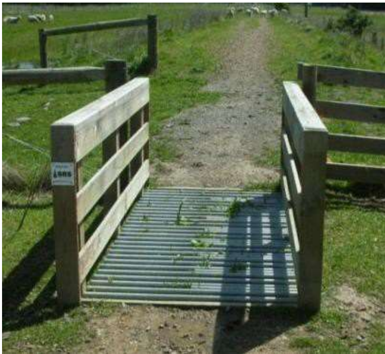
Figure 36: Cattle stop placed on straight alignment of track
