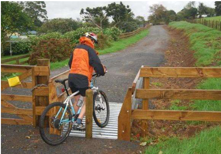
Figure 40: A central post and wing barriers help prevent motorcycle access and reduce the likelihood of stock jumping the cattle stop, but hinder accessibility for cyclists with adapted bikes or panniers (Photo: Jonathan Kennett)
