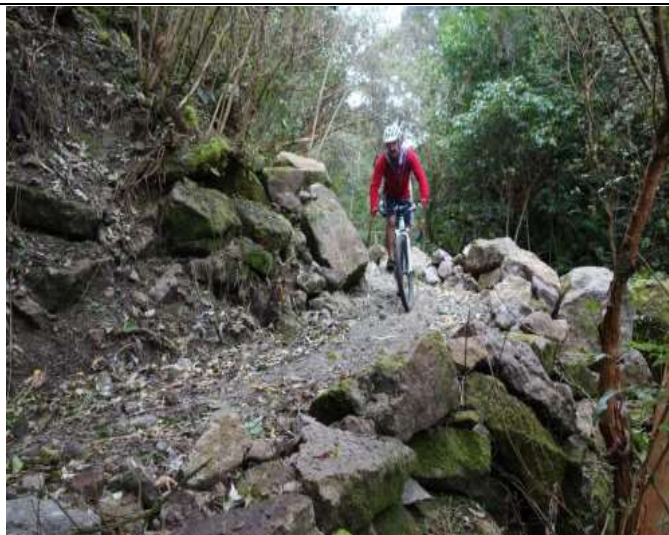
Figure E7: Rock armoured path – Nichols Creek Track, Dunedin (Photo: Kennett Brothers)
