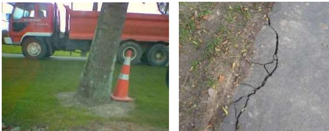
Figure B8: Heavy truck causing edge break on new pathway during construction
