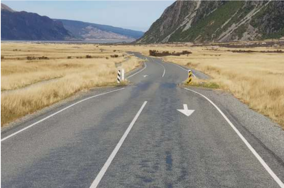
Figure 16: An example of rural traffic calming on a 60km/h road, Hooker Valley
