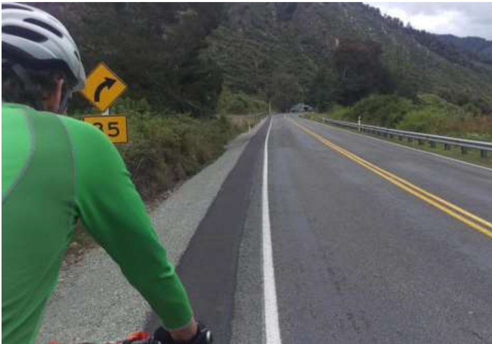
Figure 21: Smooth shoulder widening, SH6 near Murchison (Photo: Miro Kennett)
